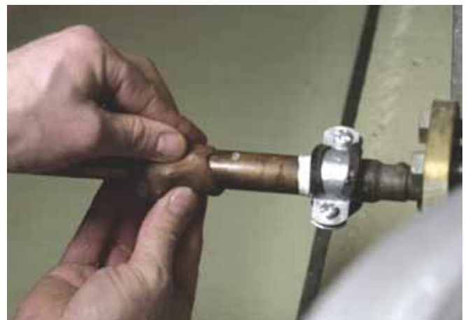
Sealing of a copper tube
